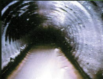
Service Water Line – Baseline Inspection
