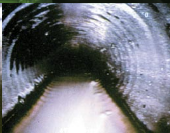
Service Water Line – Baseline Inspection
