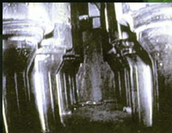
Reactor Head CRDM – Weld Inspection
